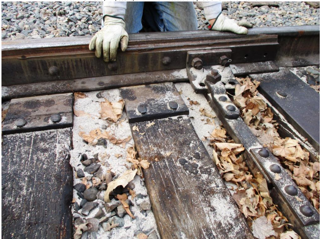
The profuse amount of sand on the switch was ruled out as the cause of its problems
