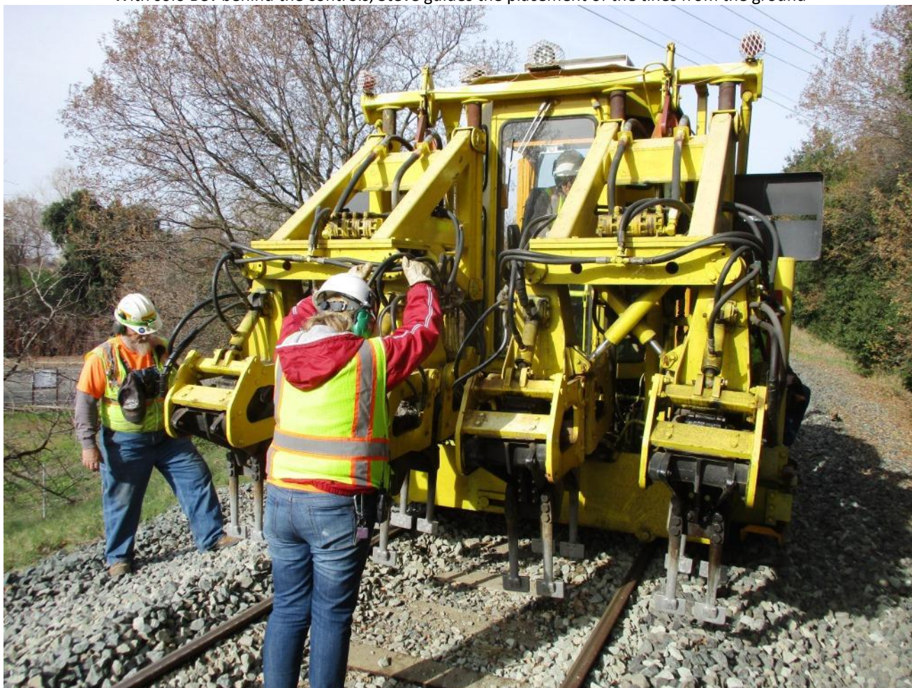
Now Steve takes the helm of the tamper as Bev guides from the ground
