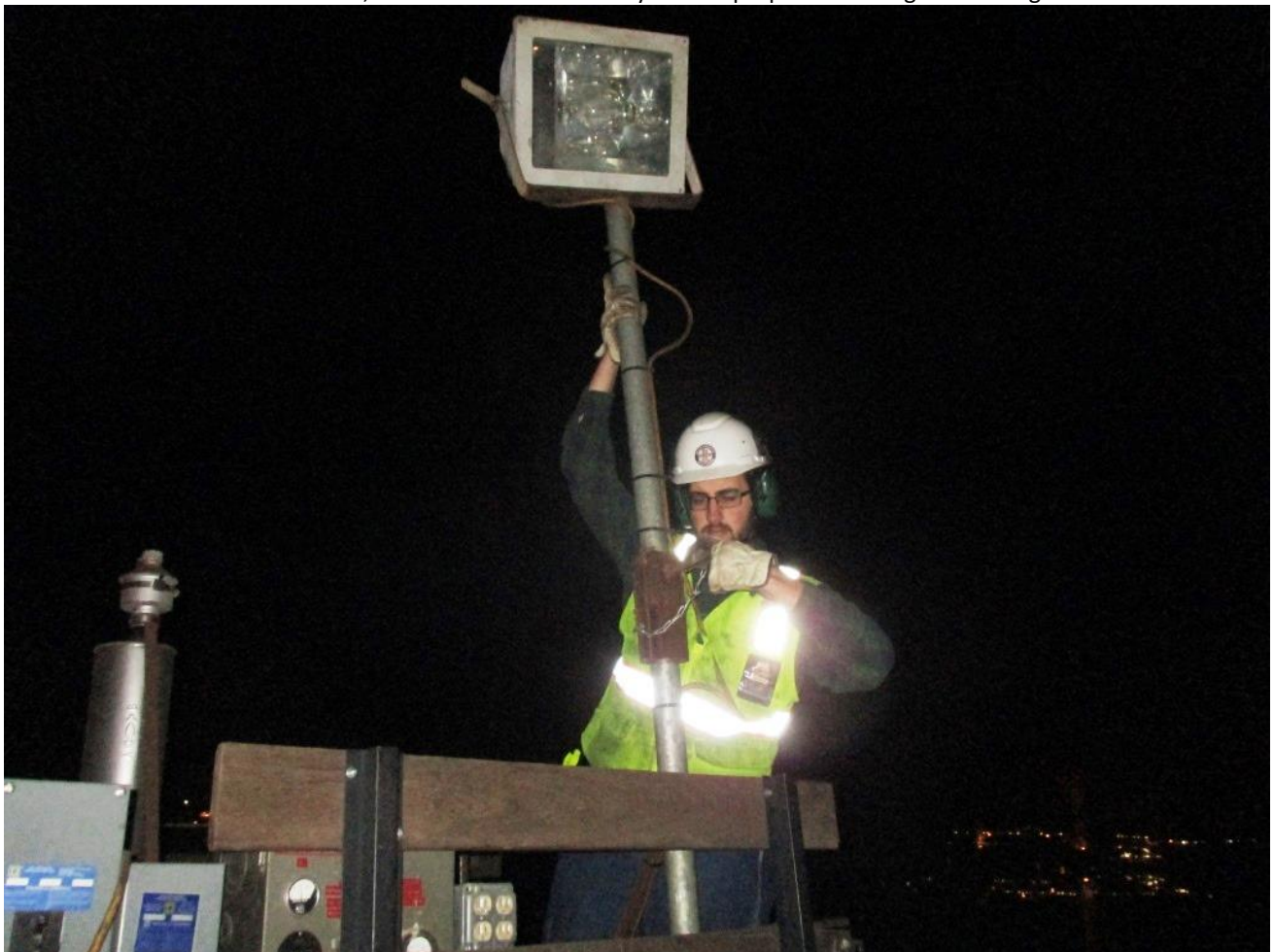
Weston sets up the light-plant
