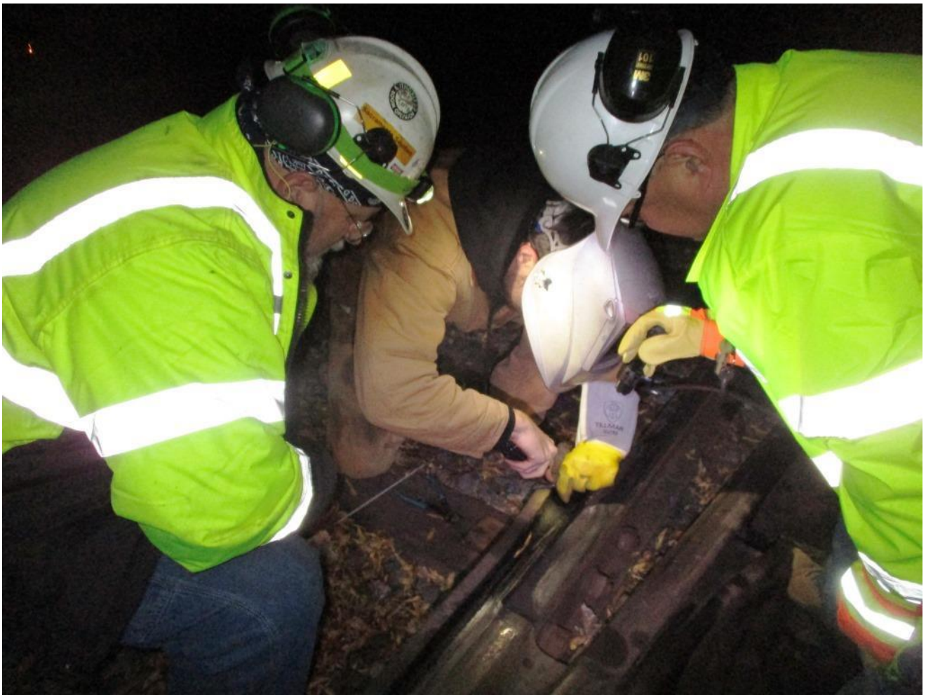
At Switch 13, Mike F. and Taka assist Kyle as he prepares the frog for welding
