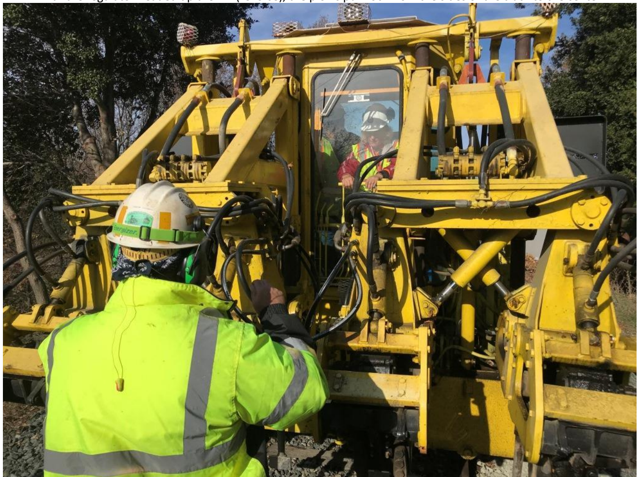
Harry in the cab with Bev provides training as Mike F. guides the operation from the ground
