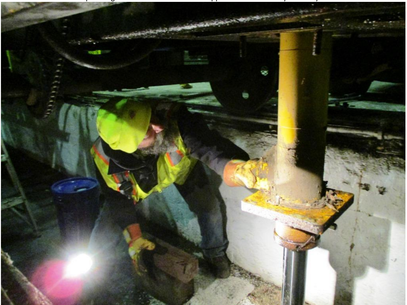
Joe, down in the pit, guides the cylinder as it is removed
