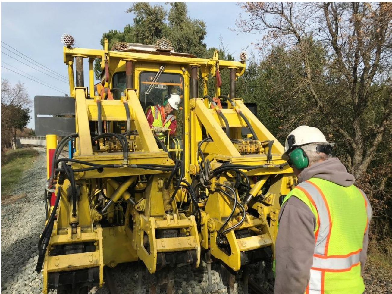
With solo Bev behind the controls, Steve guides the placement of the tines from the ground
