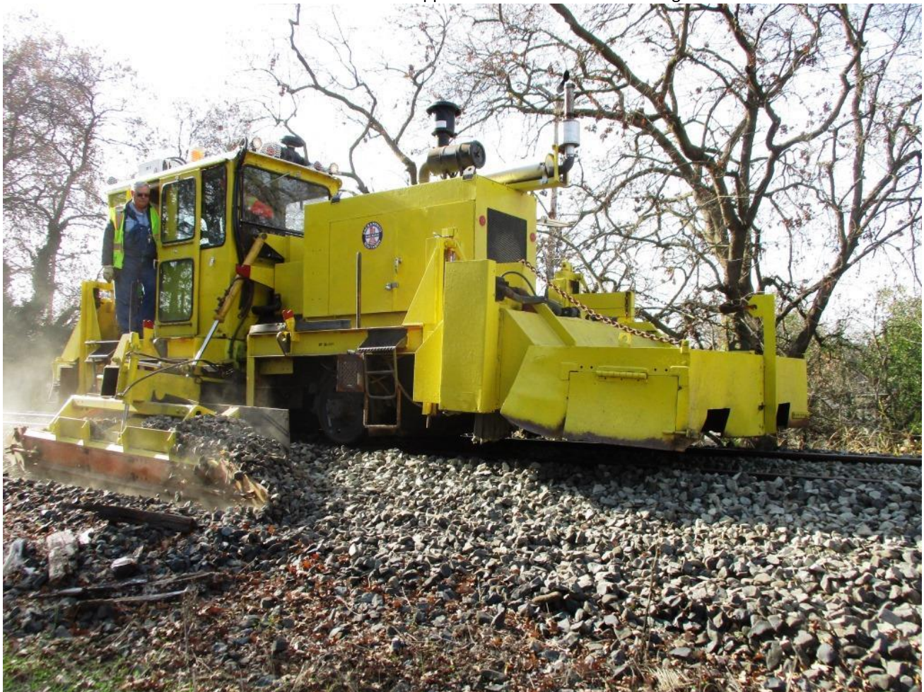
Down on the Sutterville/Zoo Line, Chris and Ed deploy the regulator's wing to pull rock up from the sides of the track onto the shoulder
