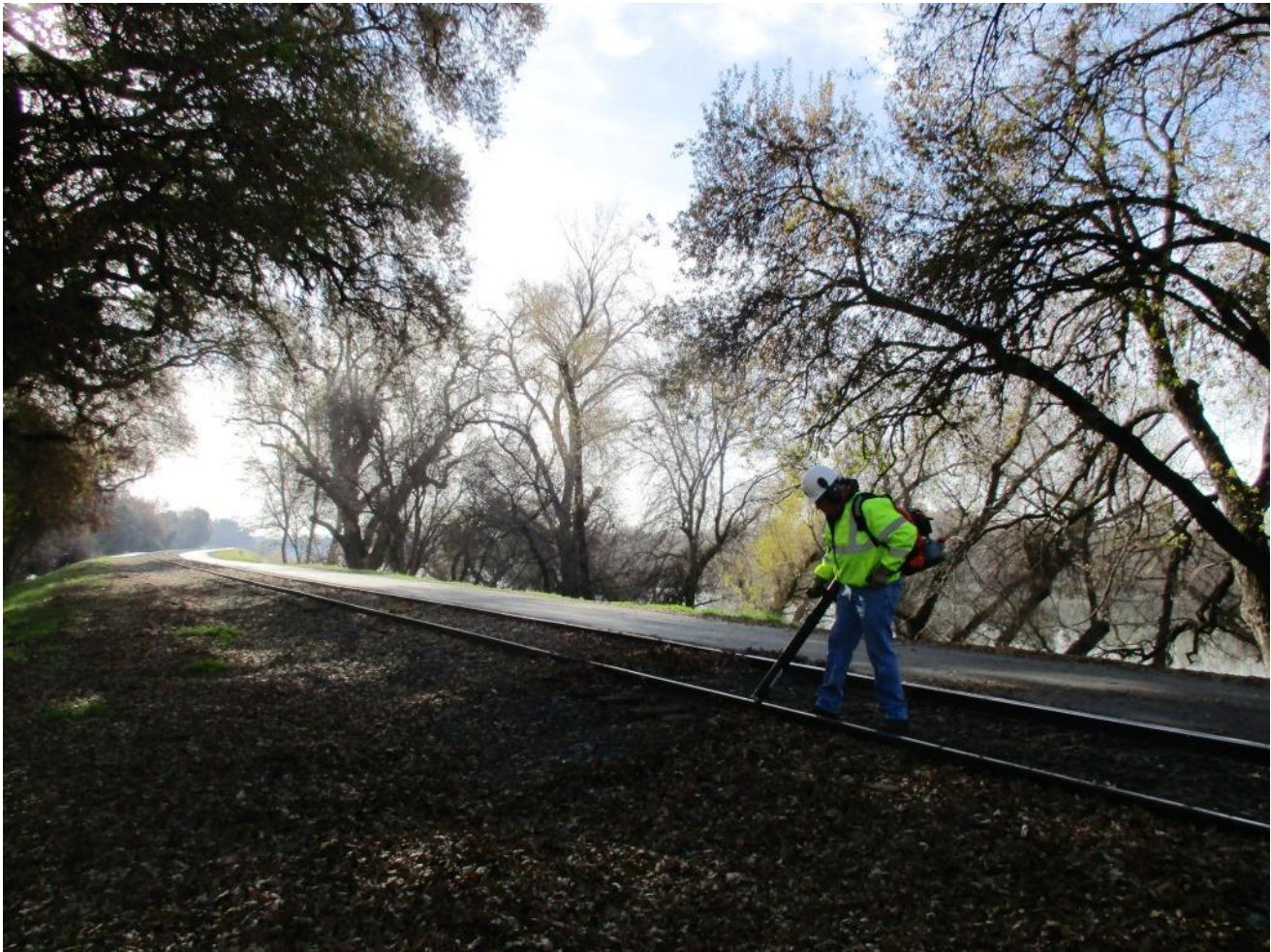
Meanwhile, Bill engages in organic debris removal at Miller Park
