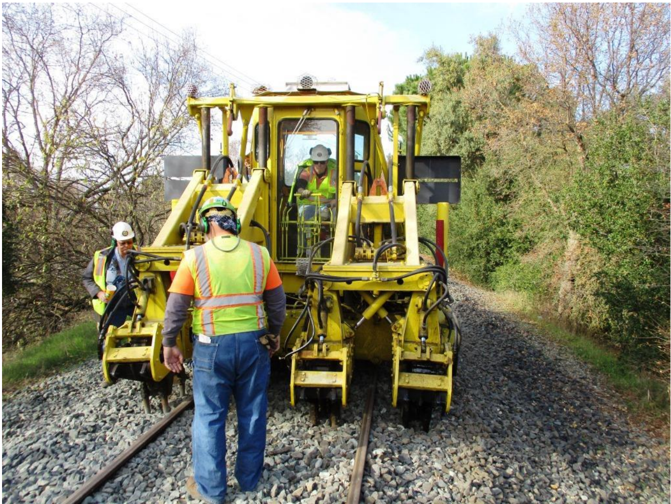
After lunch, Bill takes a turn on the tamper as Mike F. guides from the ground...
