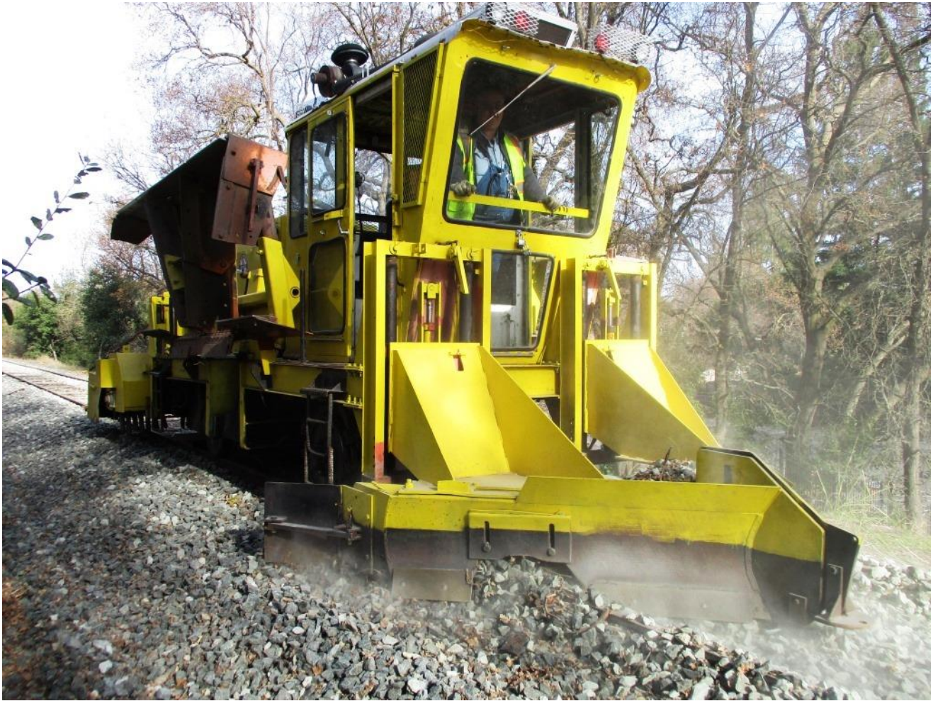
With the regulator headed up the hill (reverse), the plows pull rock from the sides of the track to the center
